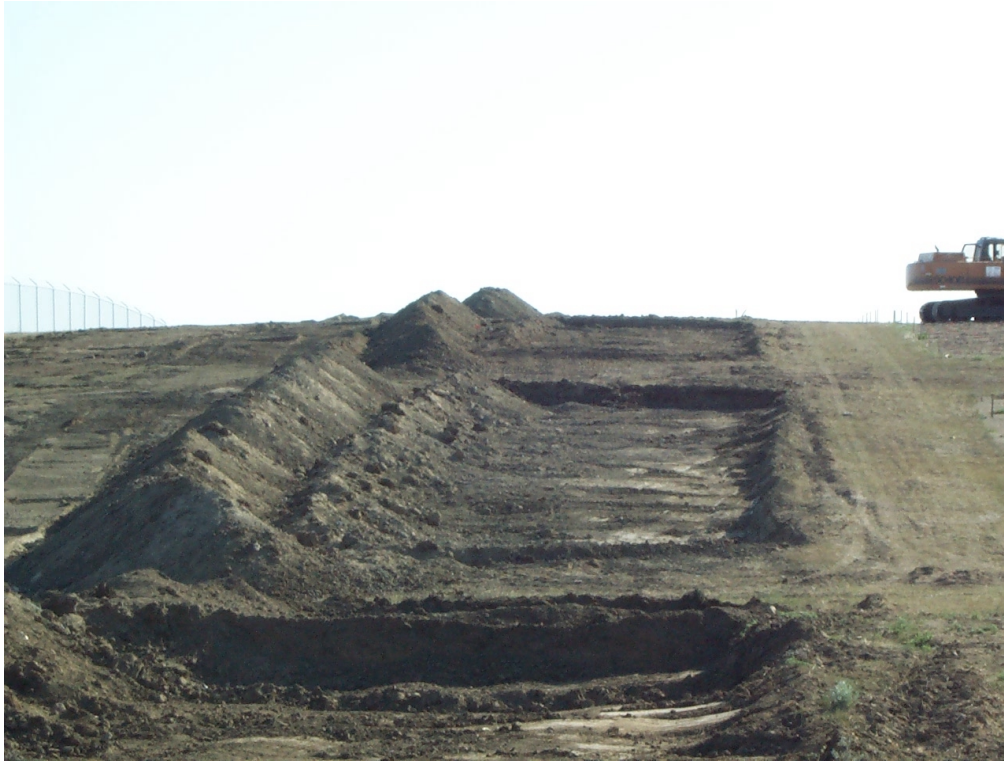
Figure 12. Range Clearance By VRL-8 Sorting Bucket
