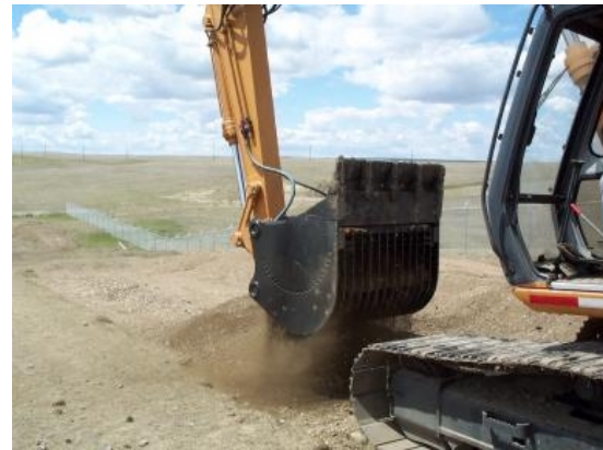
Figure A-22. VRL-8 Sorting Bucket Processing ProMac BDM48 Berm
