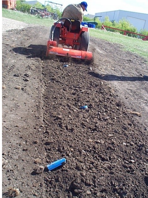
Figure 6. Garden Tractor Rototiller Bringing MRMs To The Surface
