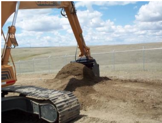
Figure A-21. VRL-8 Sorting Bucket Processing ProMac BDM48 Berm
