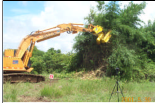
Figure 7: Debrushing Bamboo
